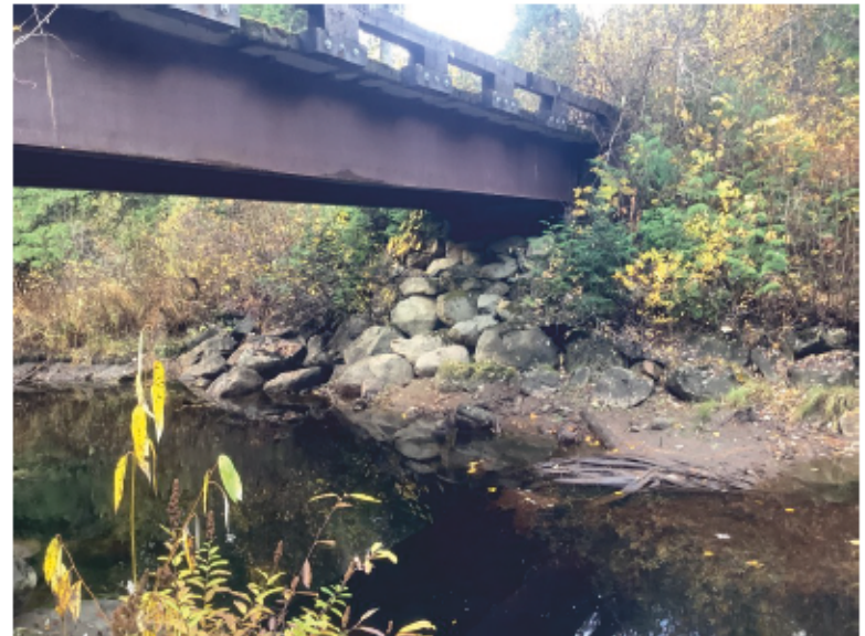
Left Bank Abutment when facing downstream
