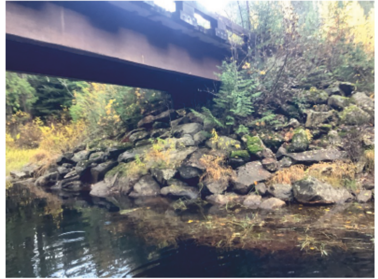
Right Bank Abutment when facing downstream
